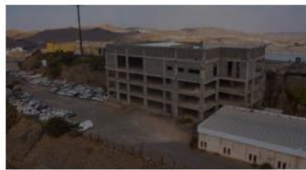
Municipal Building & Facilities 3rd Phase in ABHA
