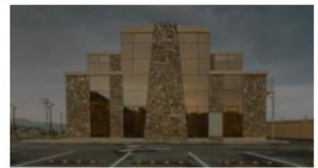
Municipal Building & Facilities 3rd Phase in Tabab Village
