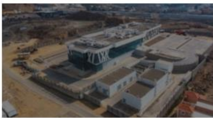
Regional Control Center for the (SEC) Electricity Company
